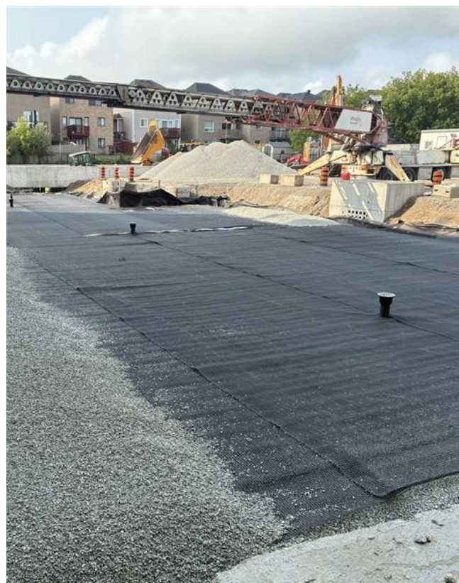
Backfill commencing on top of the tank
