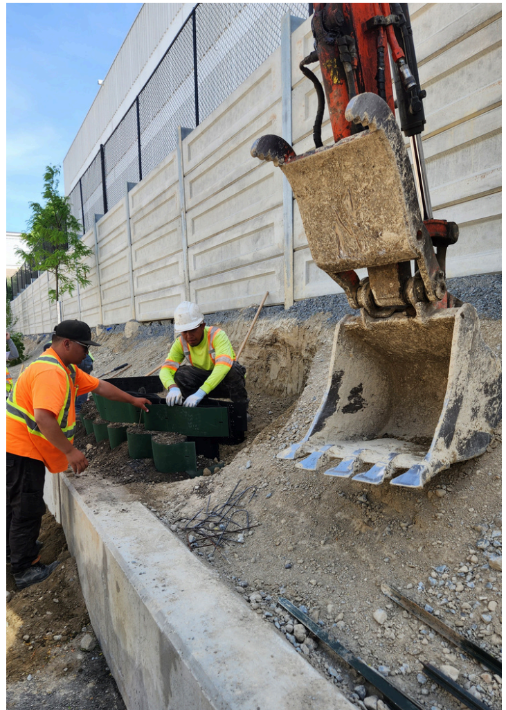
Field installation on slope
