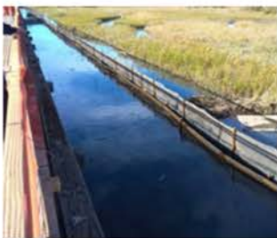
Temporary Swing Gates With E-Fence Gate Panels
