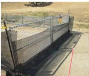
Temporary Swing Gates With E-Fence Gate Panels
