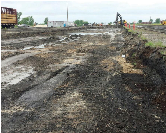
Soil conditions (pre-installation)
