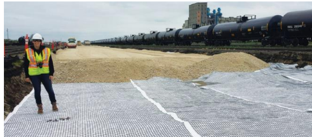
Post-installation showing Swamp Grid® soil reinforcement performance.
