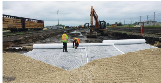
Swamp Grid® installation in progress
