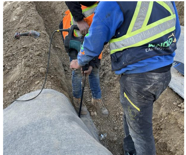
CCX-M® Being Anchored
