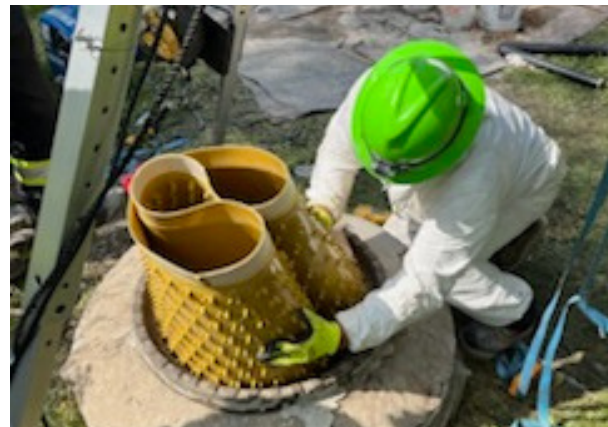
Flexliner being placed in manhole
