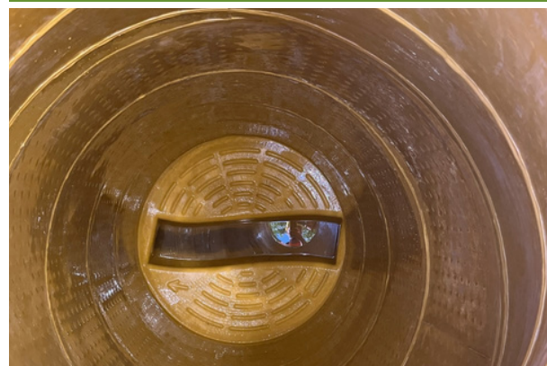
Flexliner fully installed in manhole
