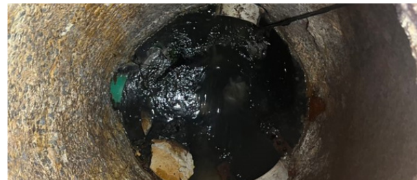
Manhole chamber before rehabilitation
