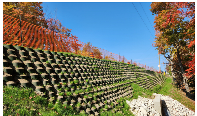
Completed Titan Earth Slope™ - Honey Comb system
