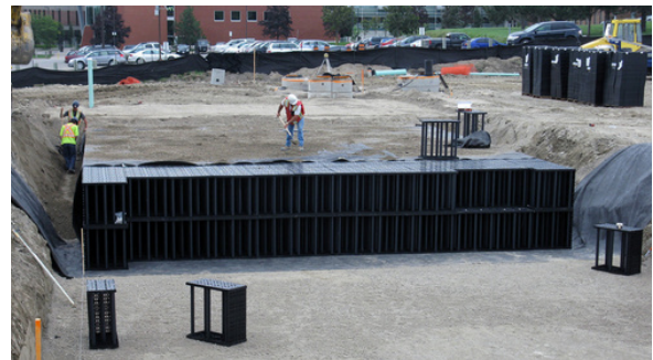
Beginning of Installation
