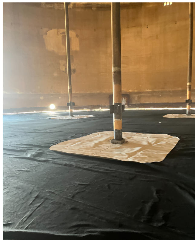
Bottom layer of geotextile
