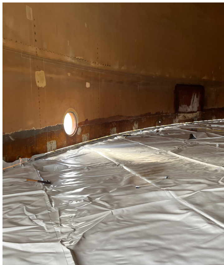
Liner attached to the tank side wall
