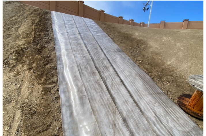
CCT1™ transversally installed.
