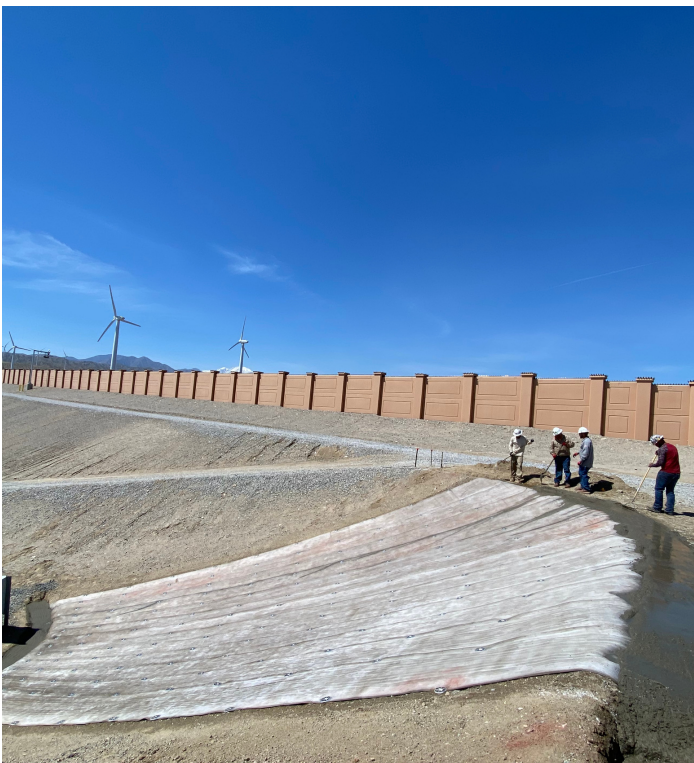
CCT1™ secured within a concrete trench.
