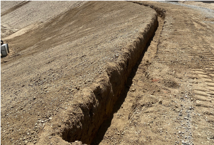
Slope regraded and anchor trench dug.
