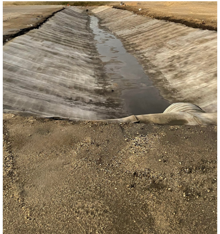
After channel lining complete.
