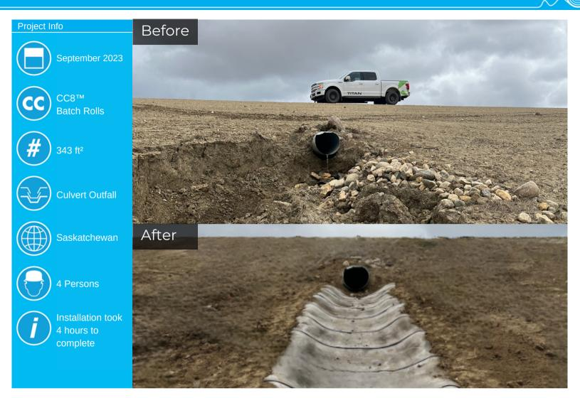
A rural municipality in Saskatchewan was seeking to solve a culvert outfall erosion problem as part of a new road construction project. Based on site conditions and needs, our team introduced <u>Concrete Canvas® (CC)</u> batch rolls as the ideal solution, which was then put into action.
