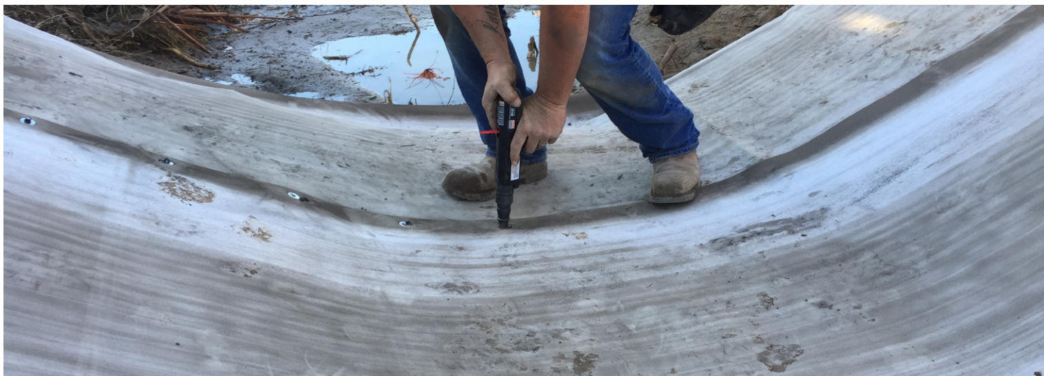
Joining of overlaps
