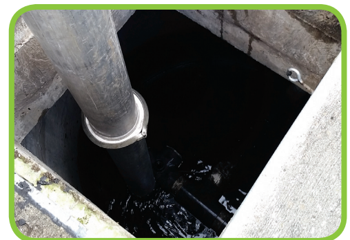
Jet Vactoring Through Access Hatch
