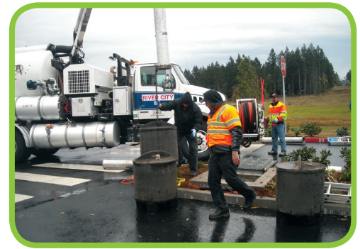
BayFilter System Cleanout
