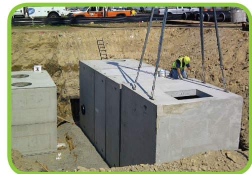
Vault End Section
