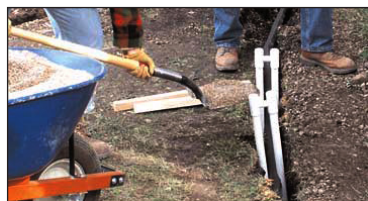
Hold the Multi-Flow in the center of the trench so that backfill can be inserted on both sides.
