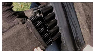
The filter is taped to the fittings to prevent sand or soil from intruding.
