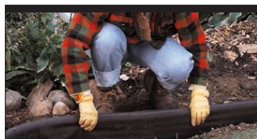
A four inch wide trench means minimal surface disruption.
