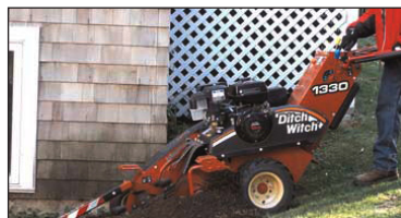
Maintaining slope during trenching is essential.
