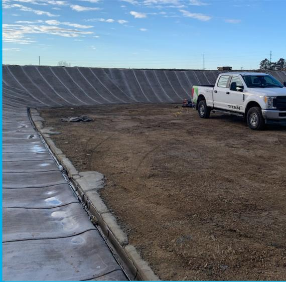
In August 2021, local contractors installed 68,864 SF (6,397m<sup>2</sup>) of Concrete Canvas® (CC5) to line berms surrounding 9 fuel storage tanks. The objective was to provide erosion protection of the berm slopes located on the fuel tank farm at a hydroelectric site.
