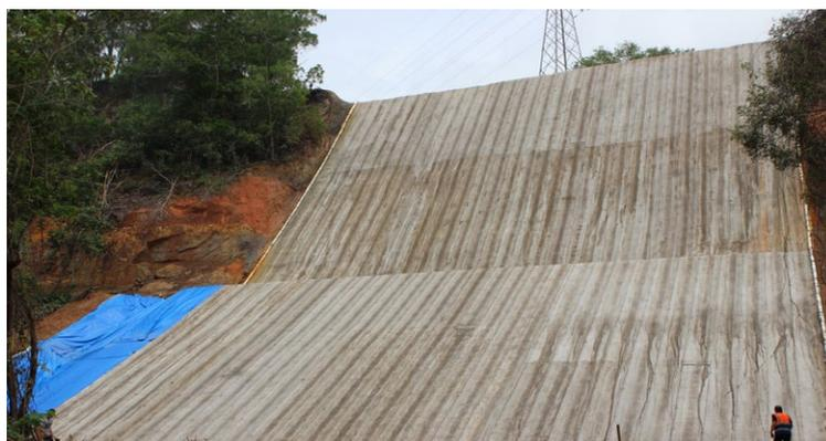
Figure 2. Typical Type I GCCM slope protection application.
