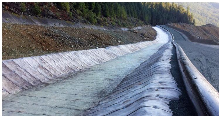
Figure 3. Typical Type II GCCM channel lining application.
