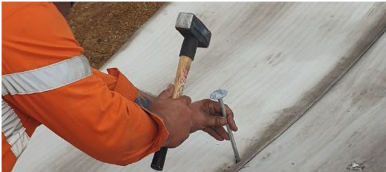
Figure 7.3 Round head peg intermediate fixing
