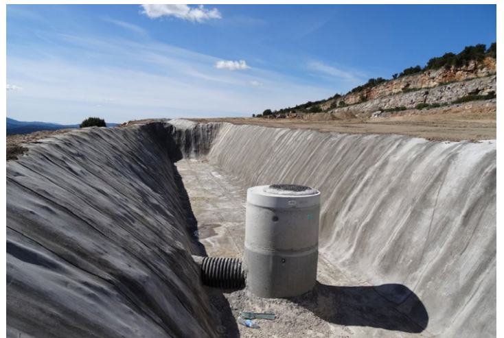
Figure 8.8 CC installed around existing infrastructure
