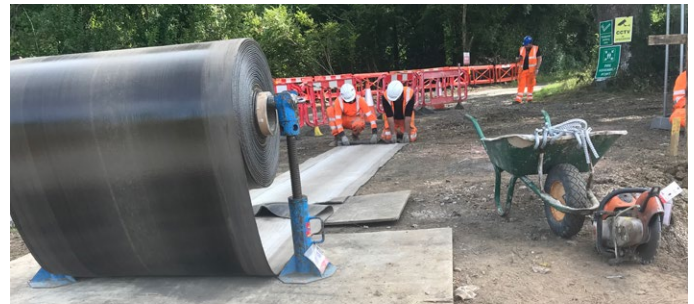
Figure 2.2 Bulk Roll dispensed from oil drum jacks
