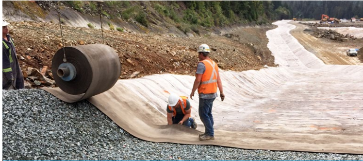
Figure 3.12 CC installed on a granular sub-drainage layer
