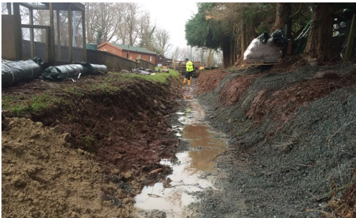
Figure 3.4 CC channel prepared with hand tools (images taken before and after install)
