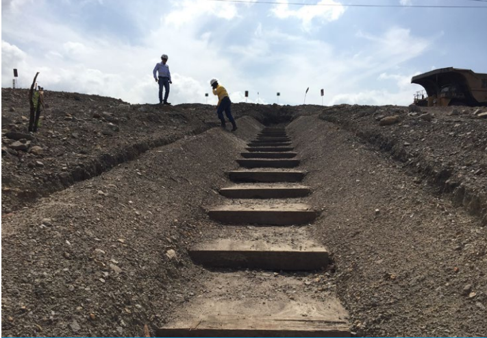
Figure 8.3 Form baffles by laying CC over structures
