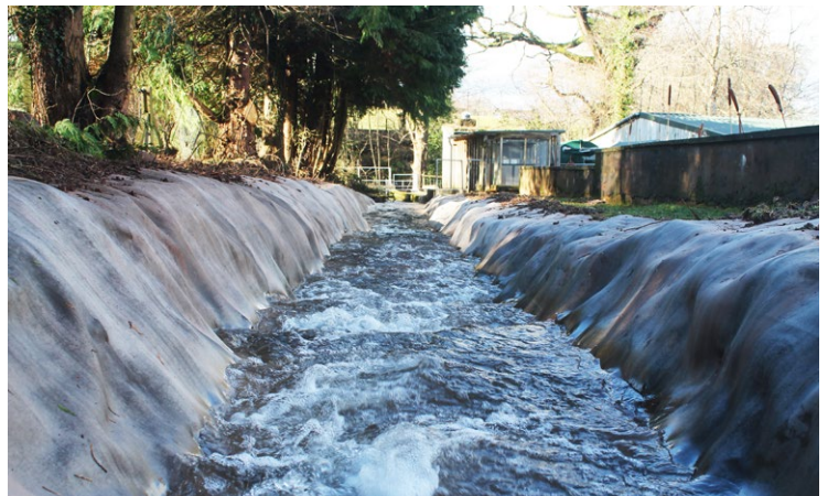
Figure 3.4 CC channel prepared with hand tools (images taken before and after install)
