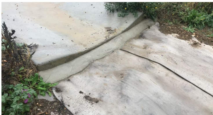
Figure 6.5 Concrete anchor trench connection
