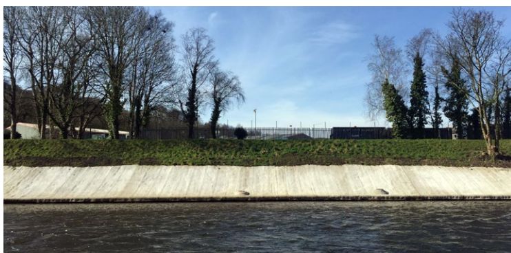
Figure 4.5 CC deployed for bank protection
