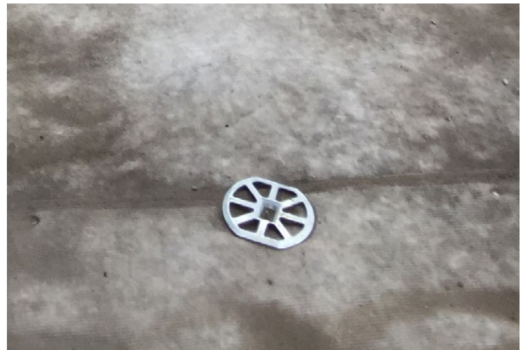
Figure 7.2 Earth percussion anchor intermediate fixing
