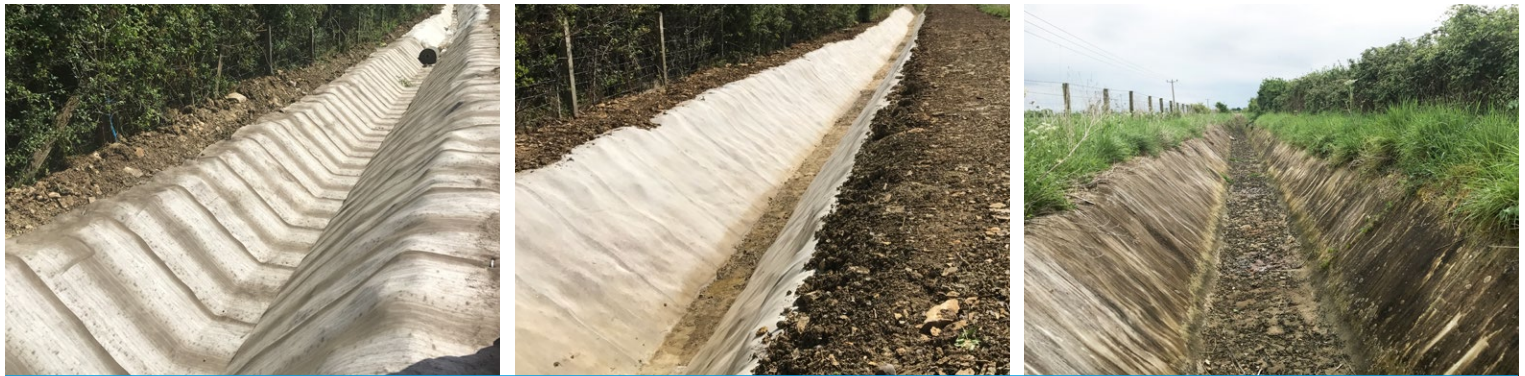
Figure 10.1 Striped surface prior to hydration, more uniform surface after hydration, darkening of surface 3 years later
