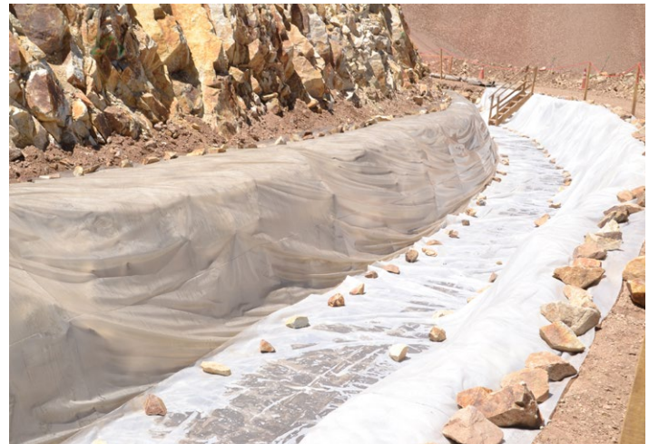
Figure 9.1 Plastic sheeting on CC during curing
