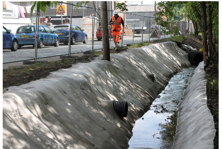
Figure 8.6 Retrospective pipe penetration
