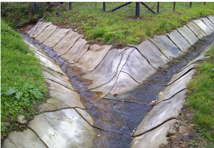
Figure 8.7 CC manipulated to form junctions
