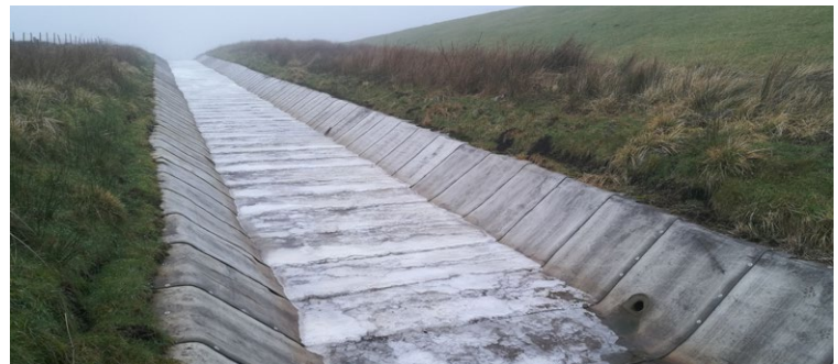
Figure 3.13 CC channel remediation
