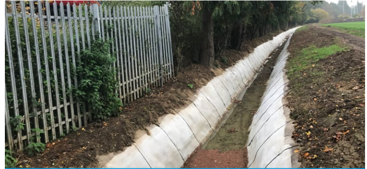
Uniform surface achieved after jet washing surface
