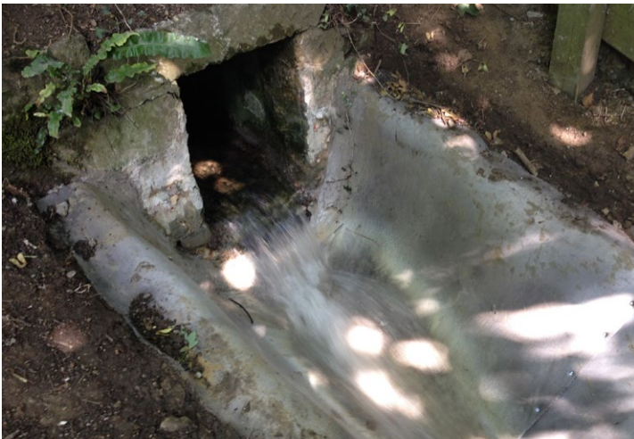
Figure 8.5 Mortar used to seal to existing infrastructure
