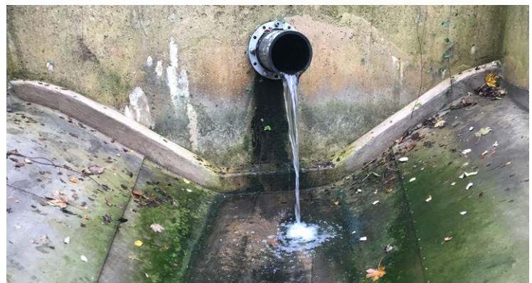
Figure 6.6 Concrete beam covering edge of CC
