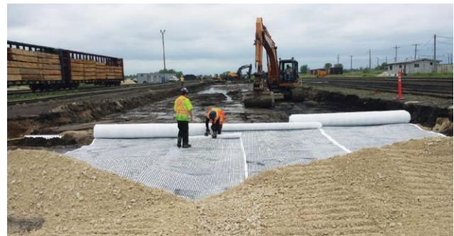
Swamp Grid™ installation in progress
