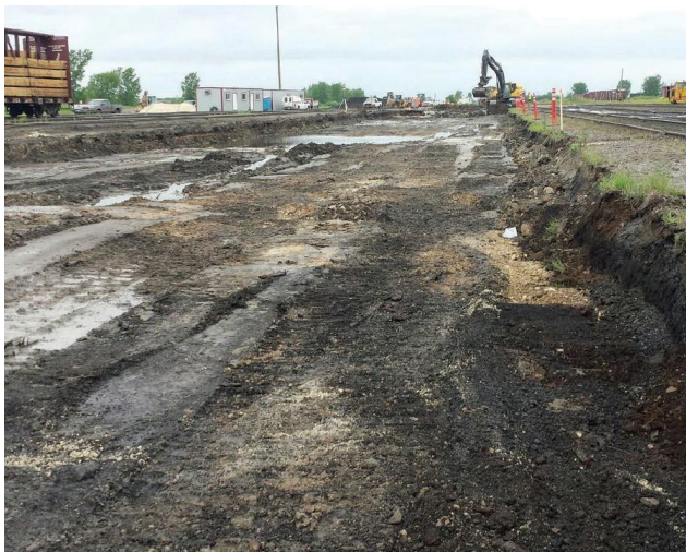
Soil conditions (pre-installation)
