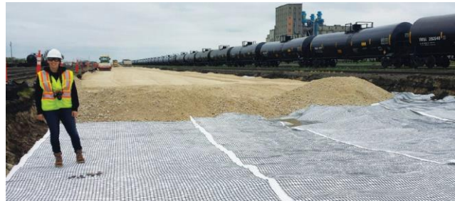
Post-installation showing Swamp Grid™ soil reinforcement performance.
