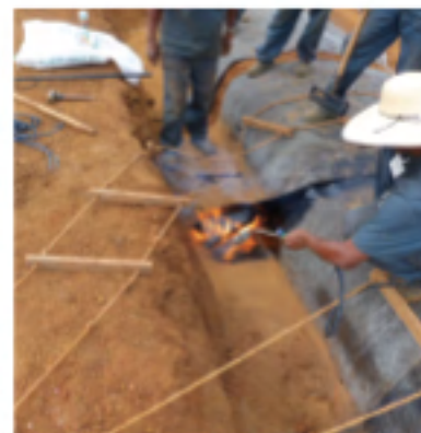
Installation in an anchor trench
