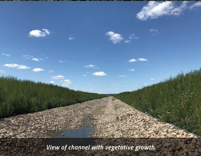
Vegetation growing through the high-performance turf reinforcement mats.
