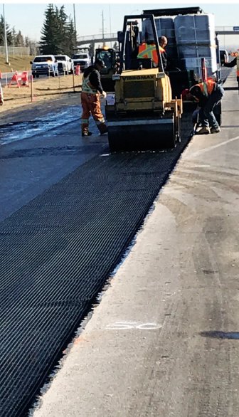
Close up of Titan’s new TE-FGP11-EPM geogrid showing desired melt of the bonding layer upon paving.
