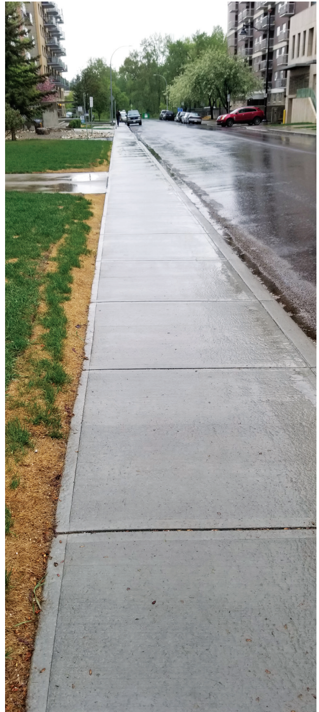
No surface cracking after 1 year.
