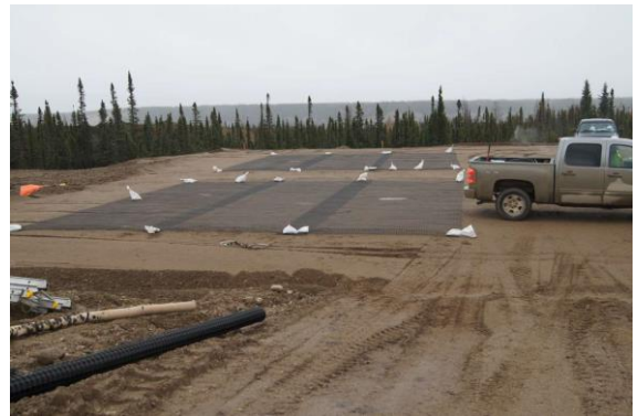
Figure 4. Laying of Horizontal Foundation Mat HFM-BL2PP
