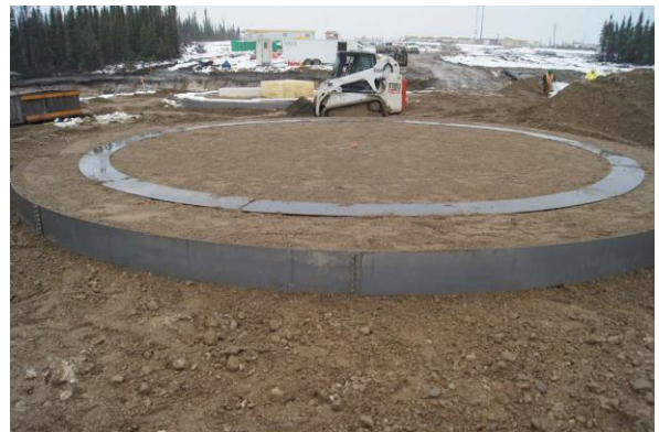
Figure 5. Construction of grade band completed and steel bearing plate installed.
