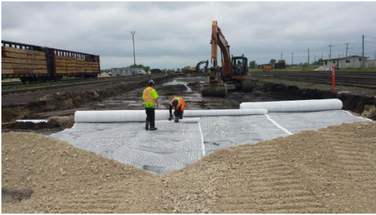
Figure 5. Granular material placed over the biaxial geogrid composite
