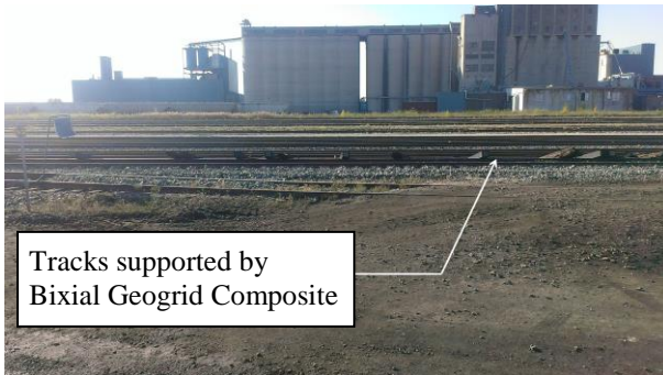
Figure 6. Completed yard in operation
