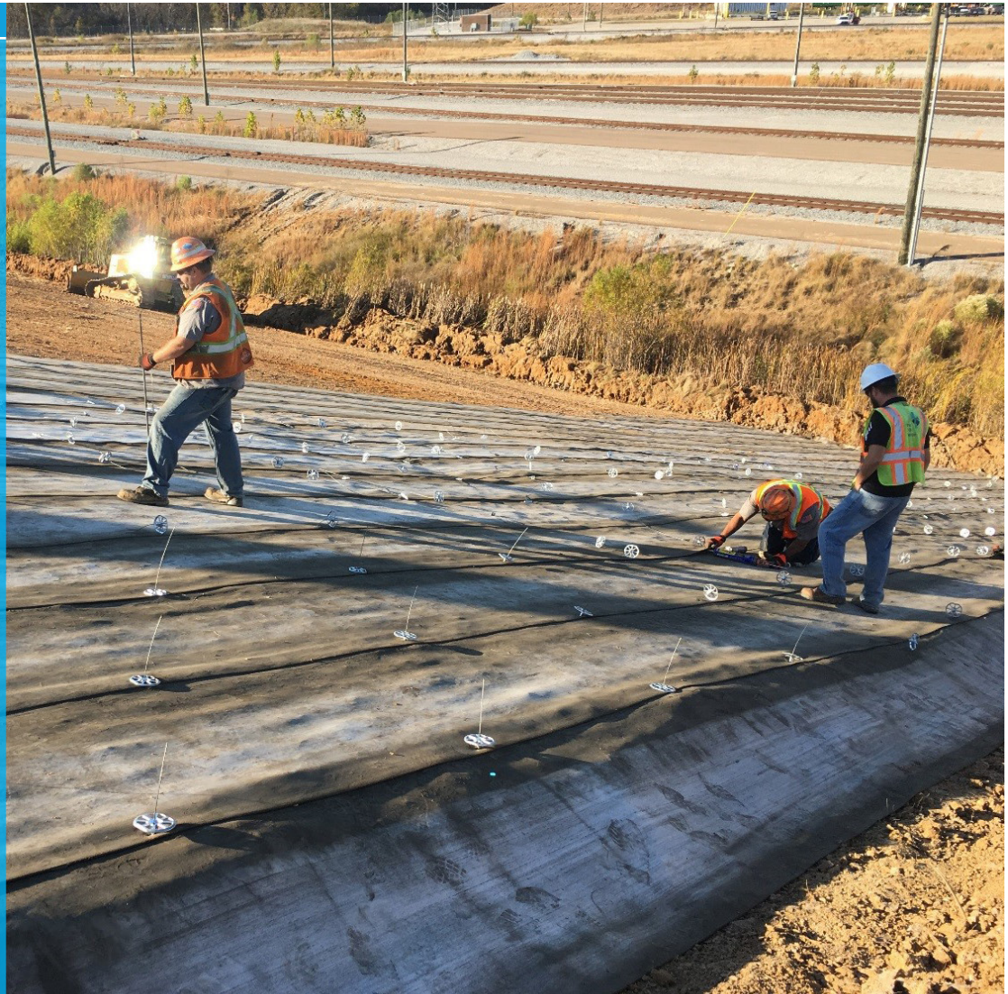
Installation of CC5 on a slope in Rossville, Tennessee
