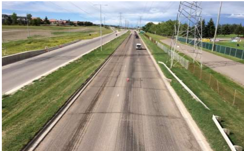
Figure 1 - General pavement condition of Sarcee Trail after cold milling of ACP
