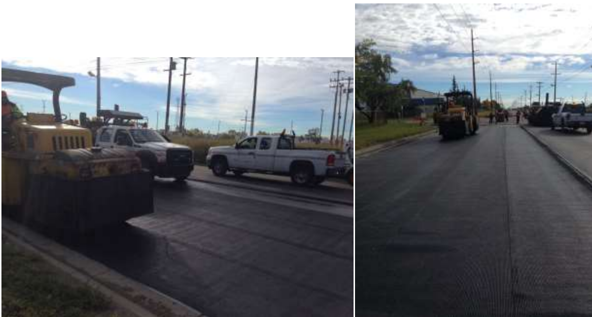
Figure 8 - 50 Ave. Grid Installation and Paving
