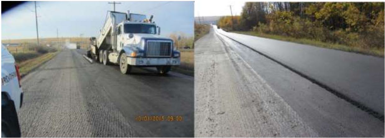
Figure 7 - 101 Street paving on Installed Grid
