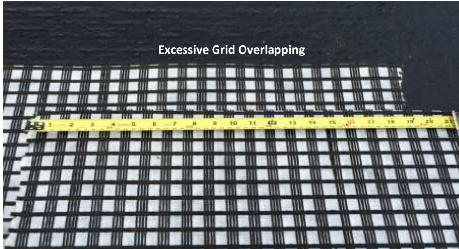
Figure 7 - 101 Street paving on Installed Grid
