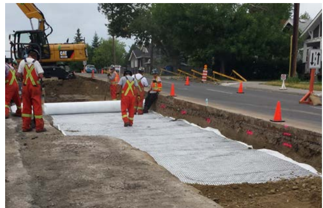
Figure 3. Laying of biaxial geogrid composite
