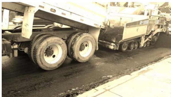
Figure 6. Placing the second lift of asphalt concrete (over the fiberglass grid).
