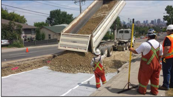
Figure 4. Placing granular subbase over the biaxial geogrid geotextile composite.
