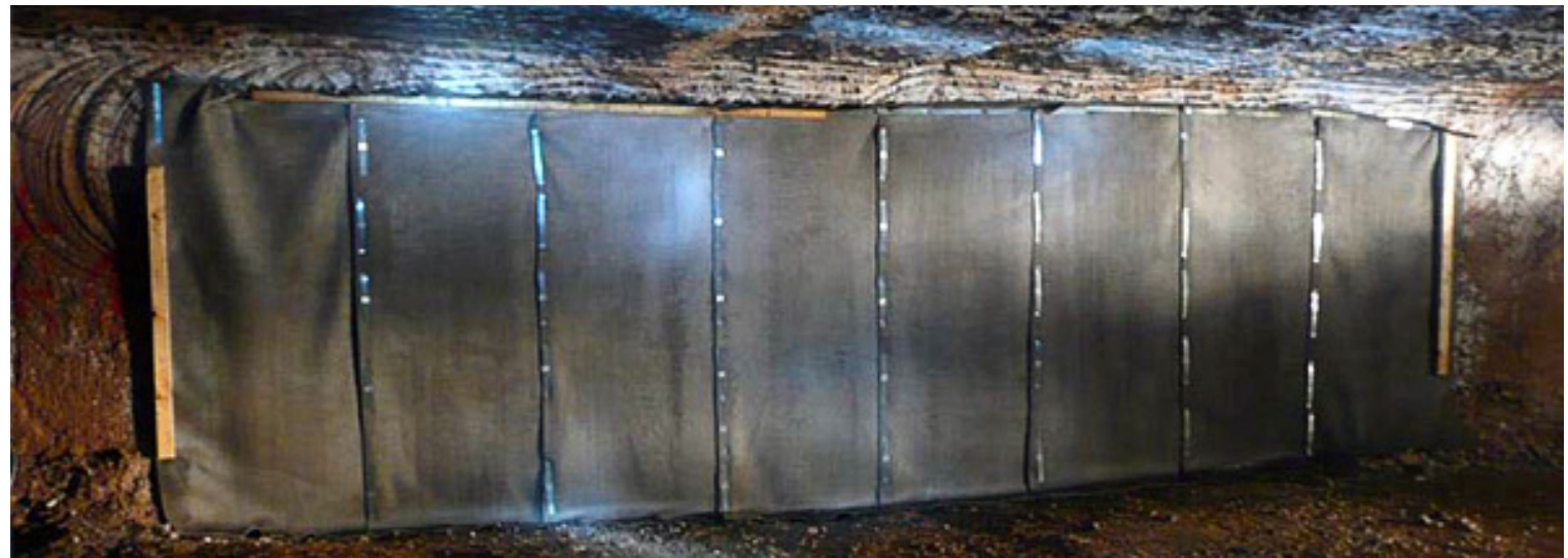
Steel bars used to support CC on another vent wall
