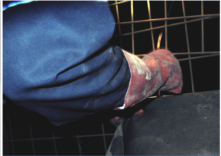
Industrial cable ties used to attach CC to wire frame
