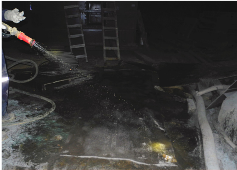
CC was hydrated before being hung and secured
