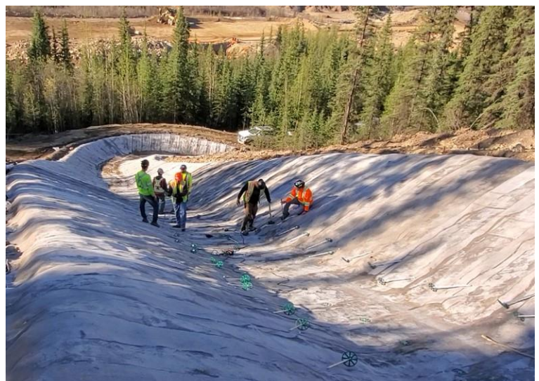
Installation of percussion anchors on emergency spillway section
