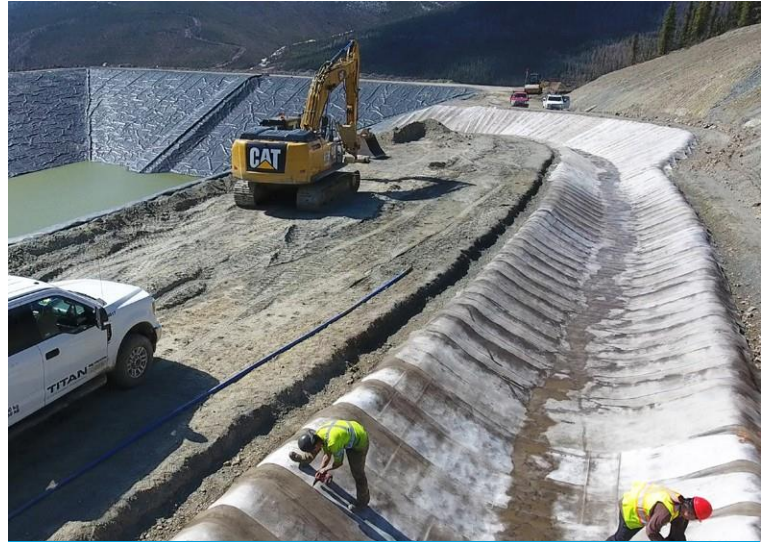
Joints were sealed and screwed for increased impermeability
