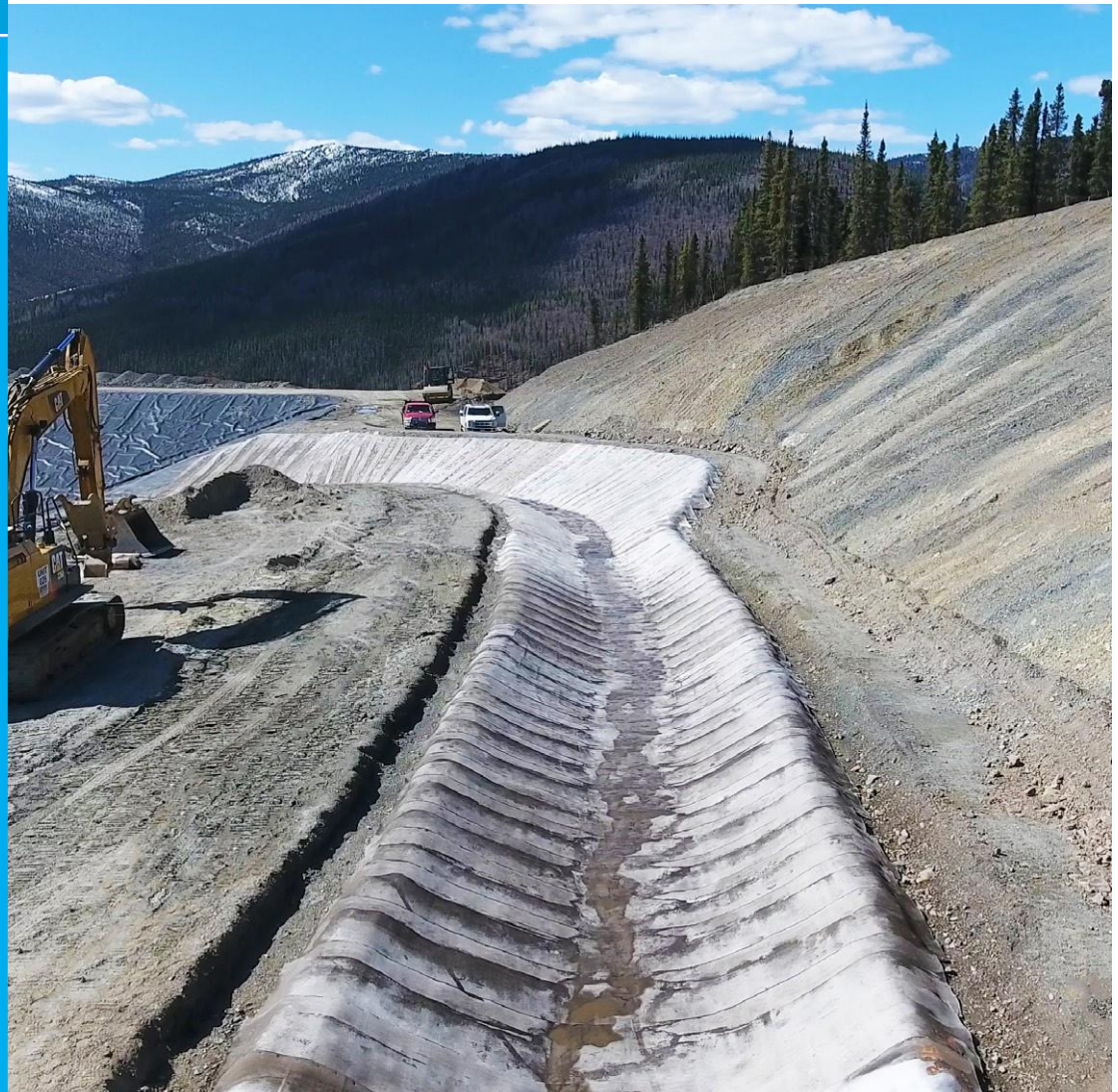
Concrete Canvas® installation at Eagle Gold Mine in Canada
