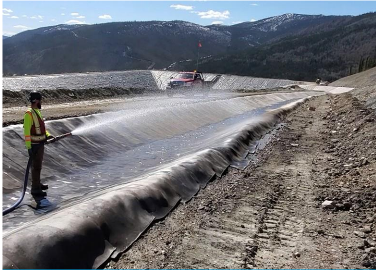
Hydration of the lined channel
