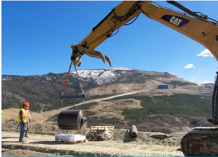
Bulk rolls of CC13 and CC8 deployed via spreader beam
