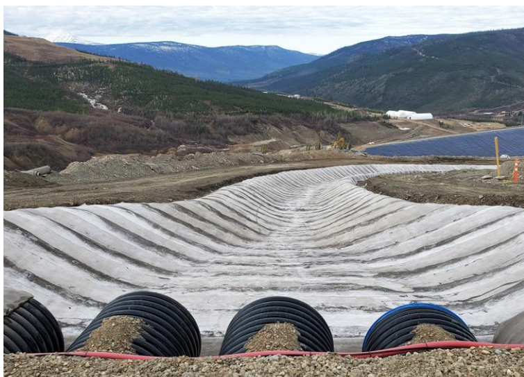
Upstream section of completed channel
