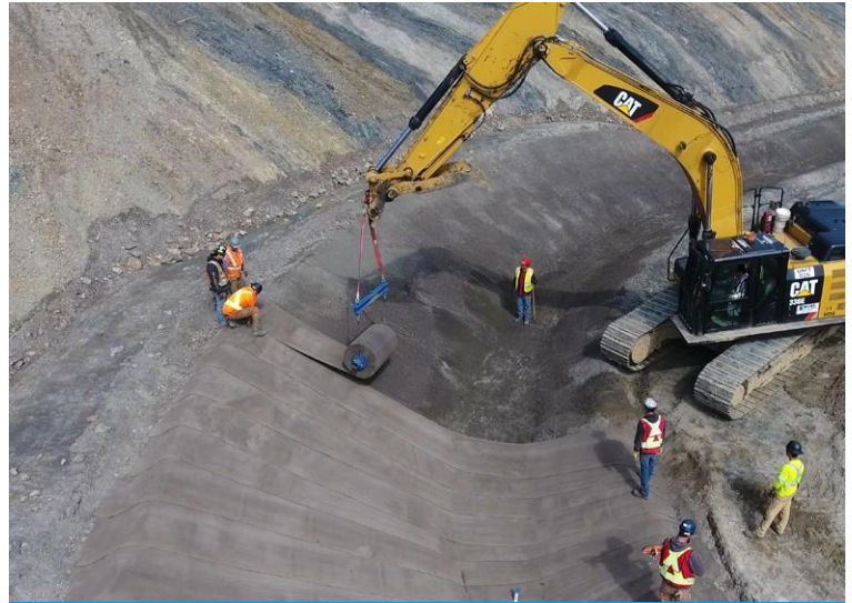
Installation starting downstream of main spillway.
