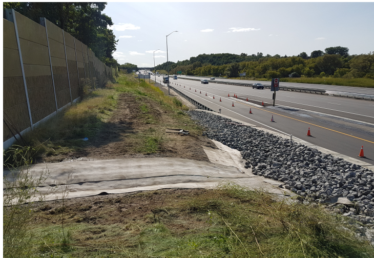
Top section joined to lower section in an L shape
