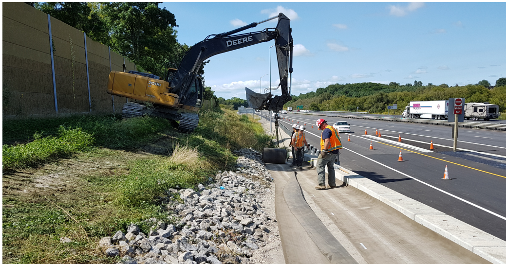
Longitudinal installation of CC
