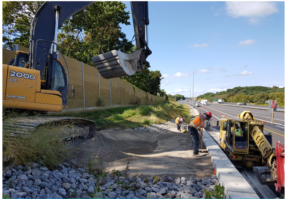
Removal of all vegetation and ground prep
