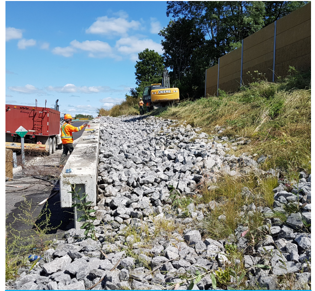
Completed rip rap placement
