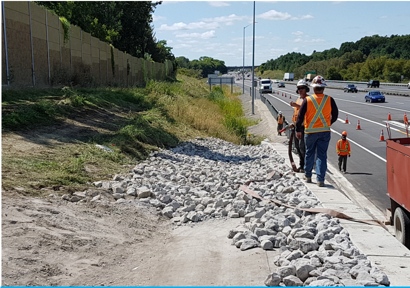
Rip Rap placed on CC prior to hydration
