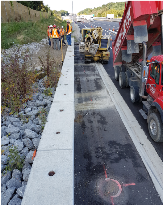
Site prior to installation
