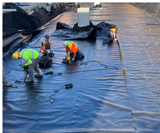
LLDPE liner installation
