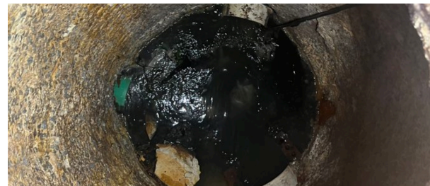
Manhole chamber before rehabilitation
