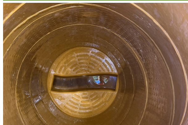
Flexliner fully installed in manhole
