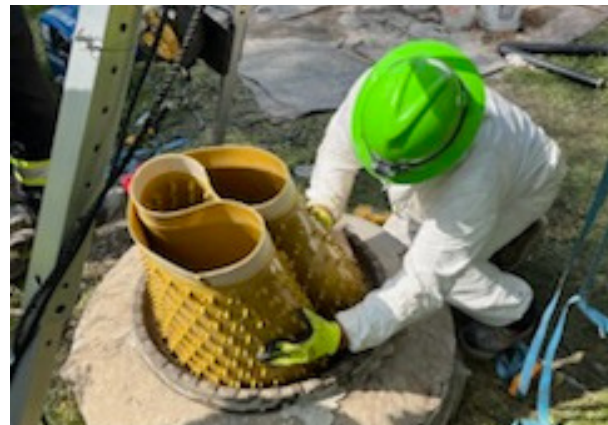
Flexliner being placed in manhole
