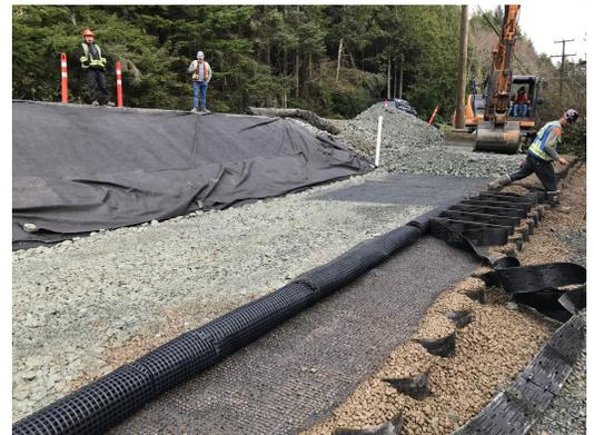
Construction of layer 1, showing Pyramid Grid and Geocell
