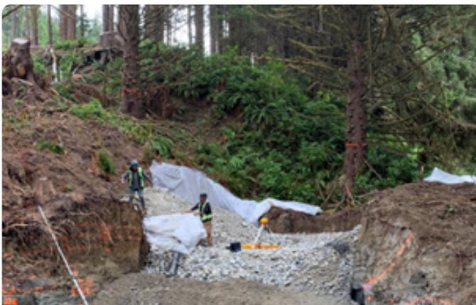
Photo illustrating the "islands" of soil left adjacent to the root systems of mature trees prior to installation of the GRS geogrid
