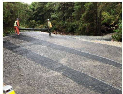
Illustration of the uniaxial geogrid in the buttress.
