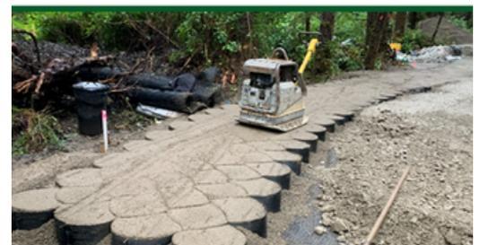
Photo illustrating typical wall construction.
