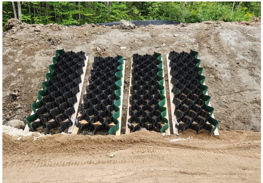
Installed system pre-vegetation
