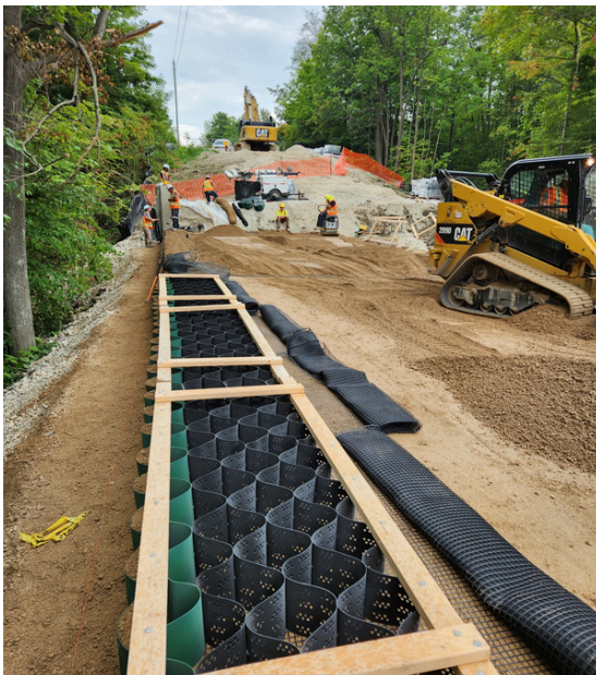
Installation in progress
