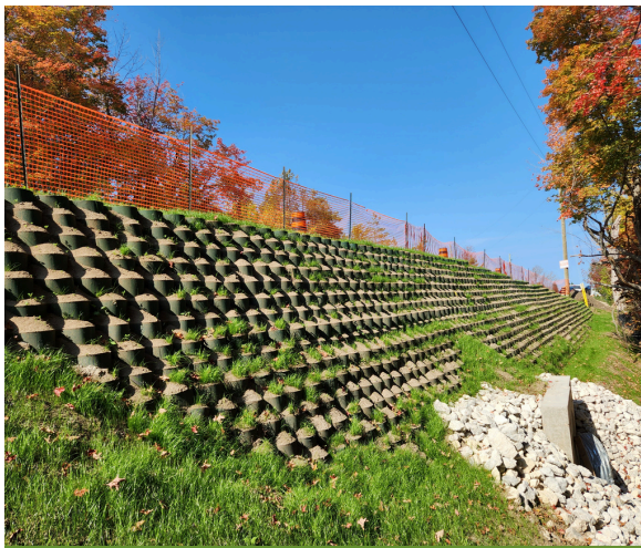
Installed system pre - vegetation growth
