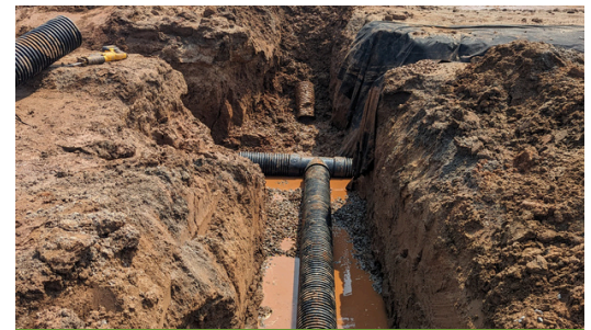
Perimeter trench with HPDE Pipe
