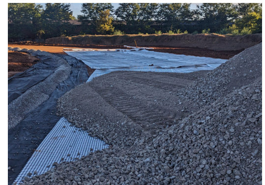
Aggregate post Swamp Grid™ installation
