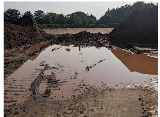
Subgrade at east end of the facility pre-installation
