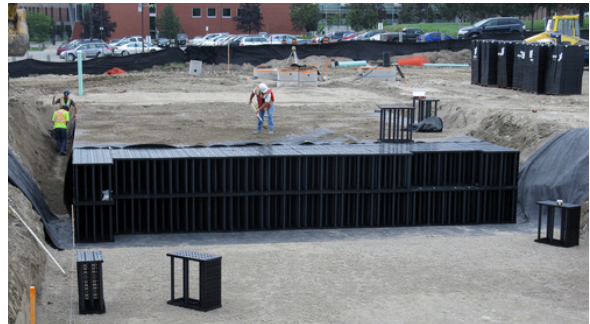
Beginning of Installation
