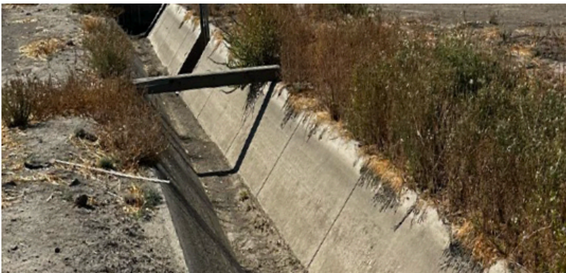
Site prior to installation
