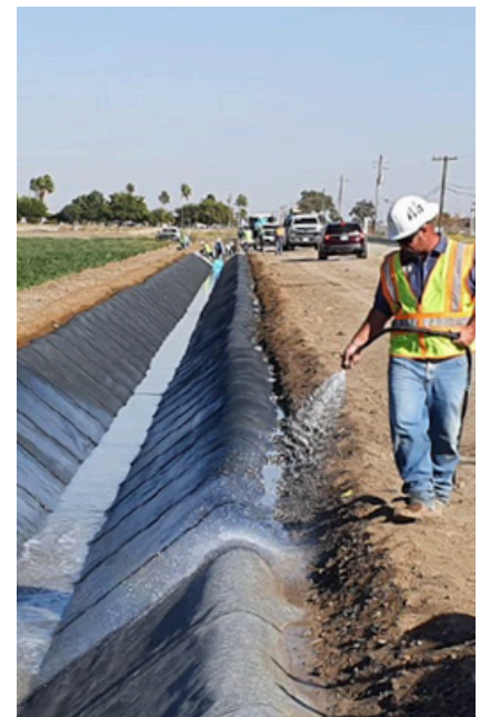
CCX™ hydrated using hose and water truck
