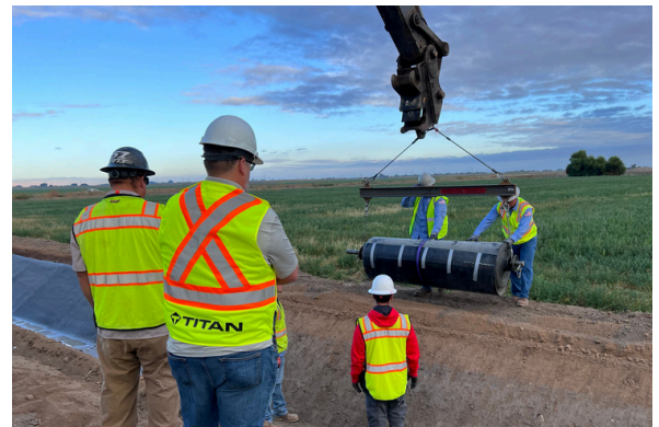
CCX™ deployed transverse using an excavator and spreader beam
