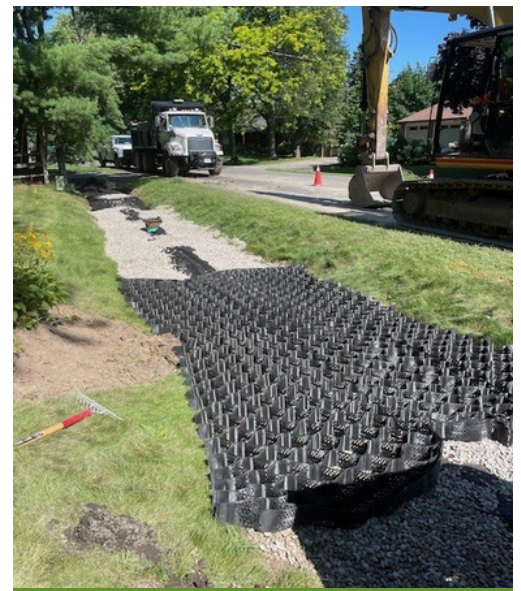
Geocell Panel Installation
