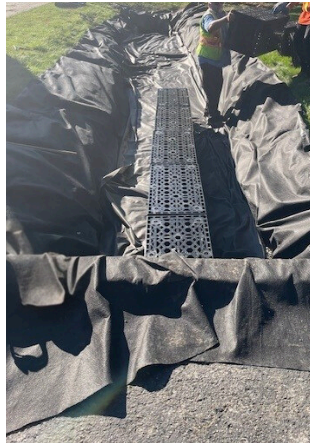
Installation of Brentwood StormTank®
