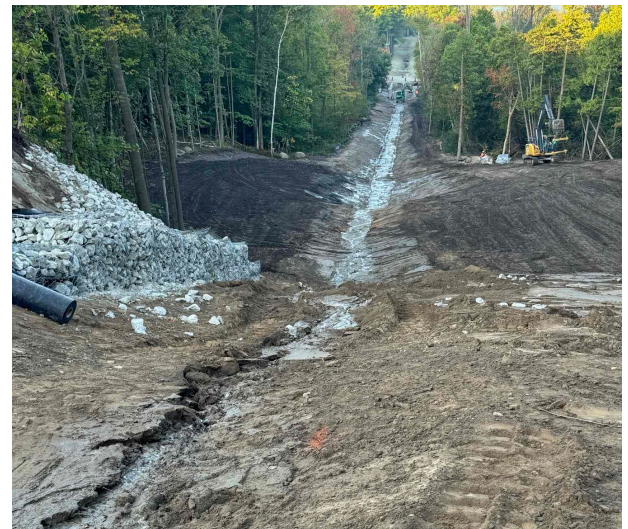
Channel before project completion.
