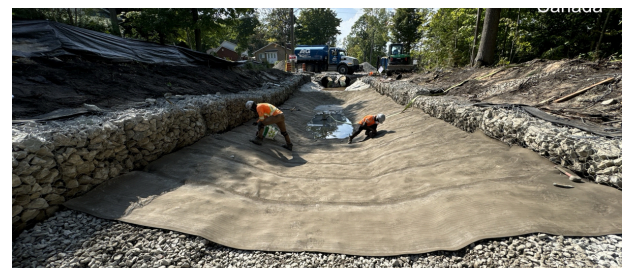
CC installation in progress.
