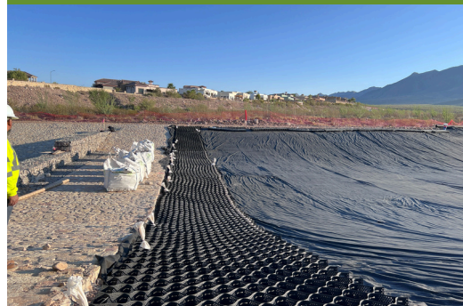
Geocell Installation
