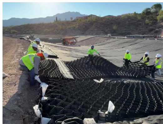
Geocell Installation
