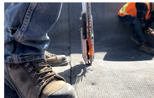
Jointing with an auto-feed screwdriver
