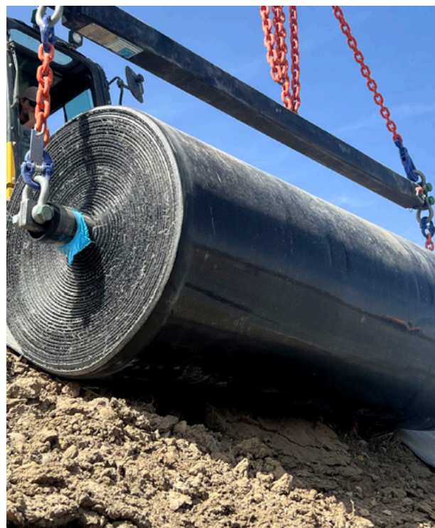
CCX-M® deployed using a spreader beam.
