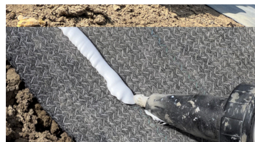
Applying an 8mm bead of adhesive sealant
