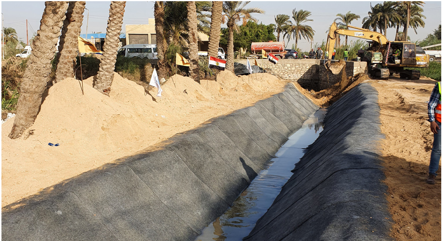
Completed installation of CCX-B following final hydration™
