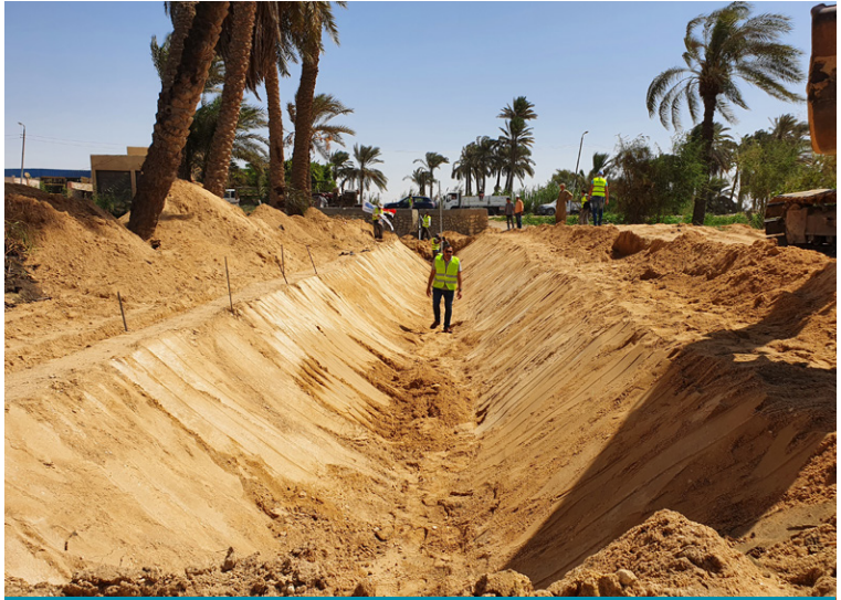
Canal profile following compaction of substrate
