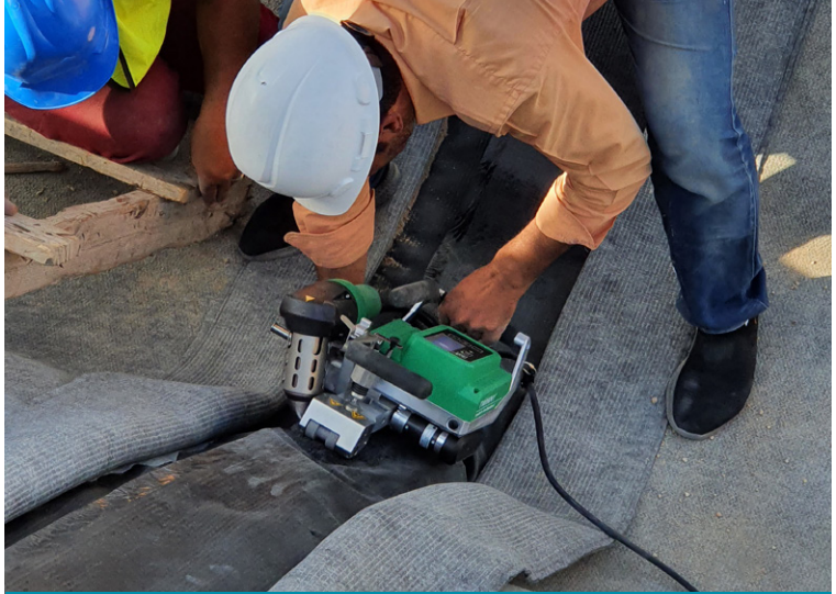
Thermally welding geomembrane backing layers
