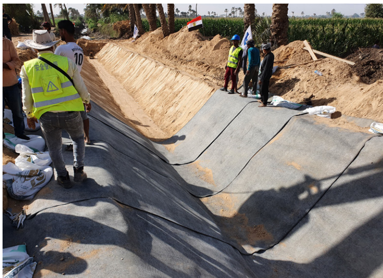
Layers of CCX-B™ overlapped by 100mm
