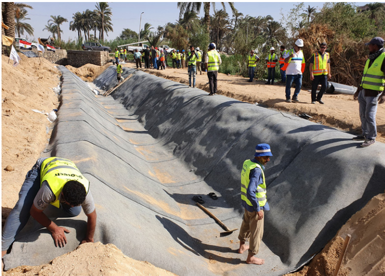
Tucking downstream edge into anchor trench
