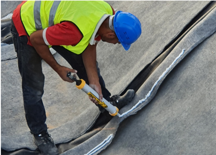
Adhesive sealant applied to overlaps
