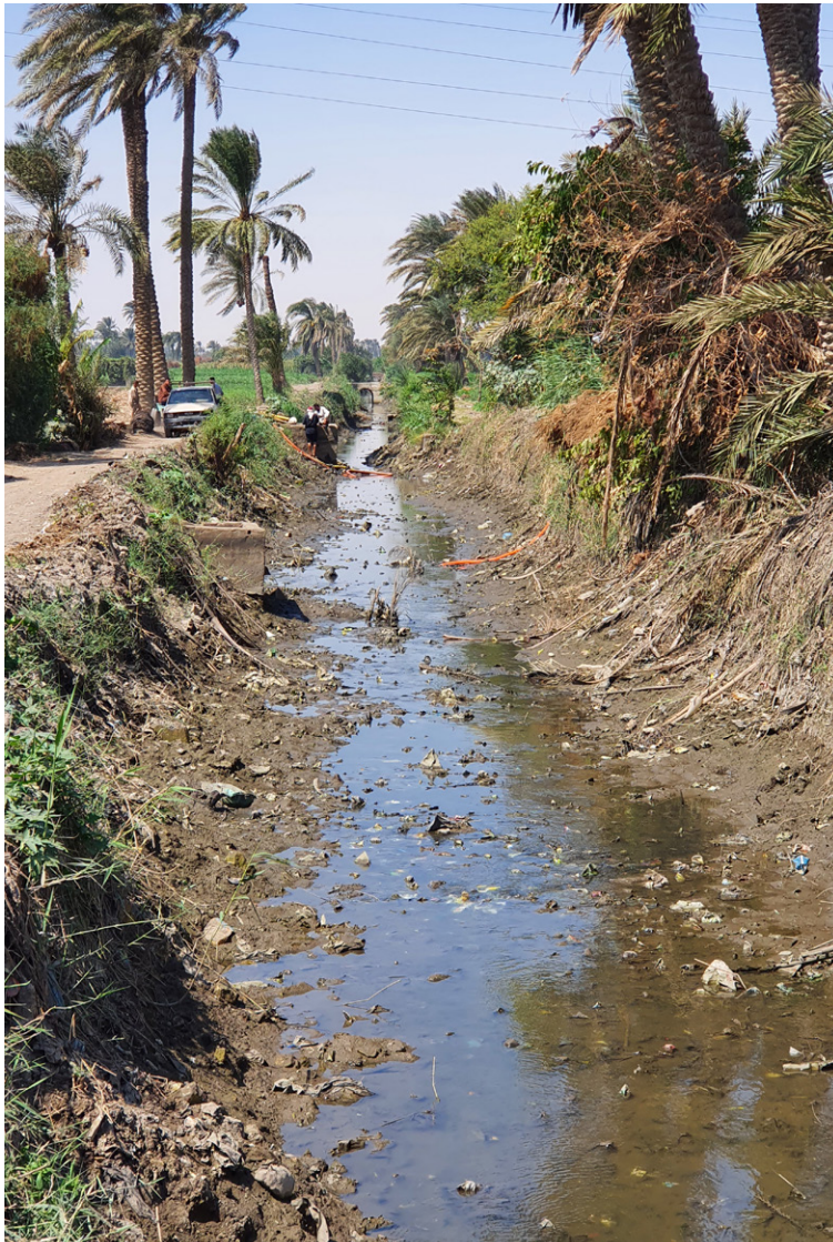
Site prior to works
