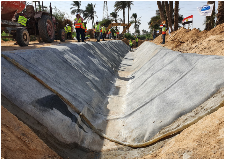
Downstream anchor trench backfilled with poured concrete
