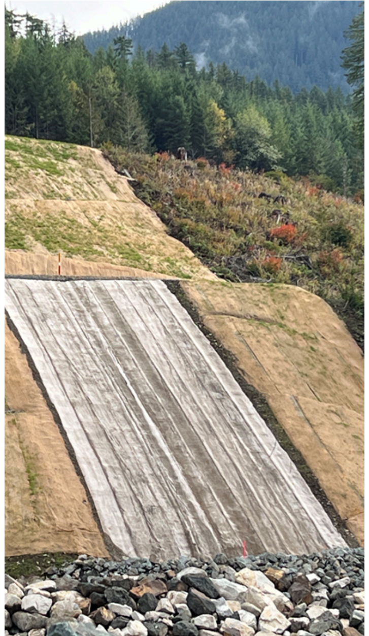
After CCT2™ Installed
