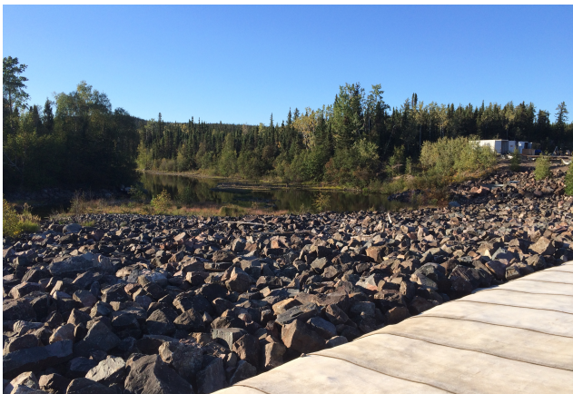
Rip rap placed to dissipate water flowing over weir
