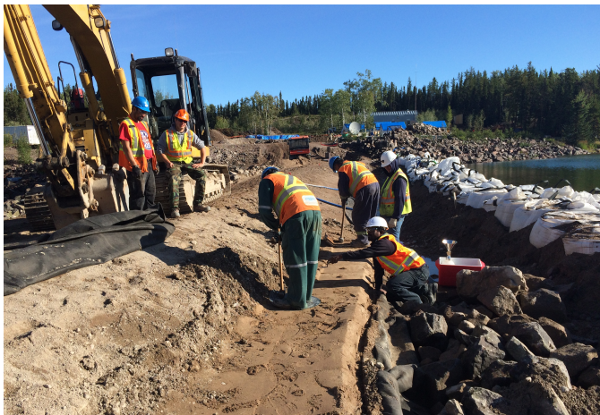
Limited working area on site
