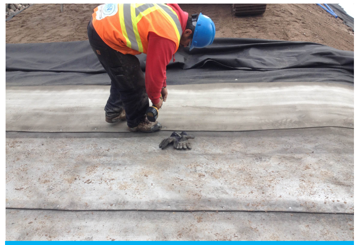
Securing overlapped CC joints
