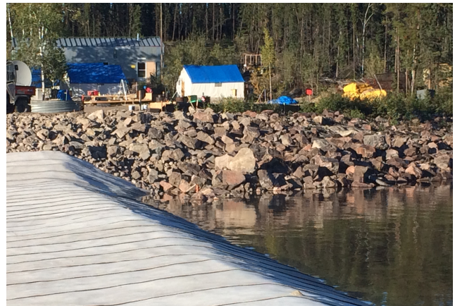
Completed weir -looking towards the lake side
