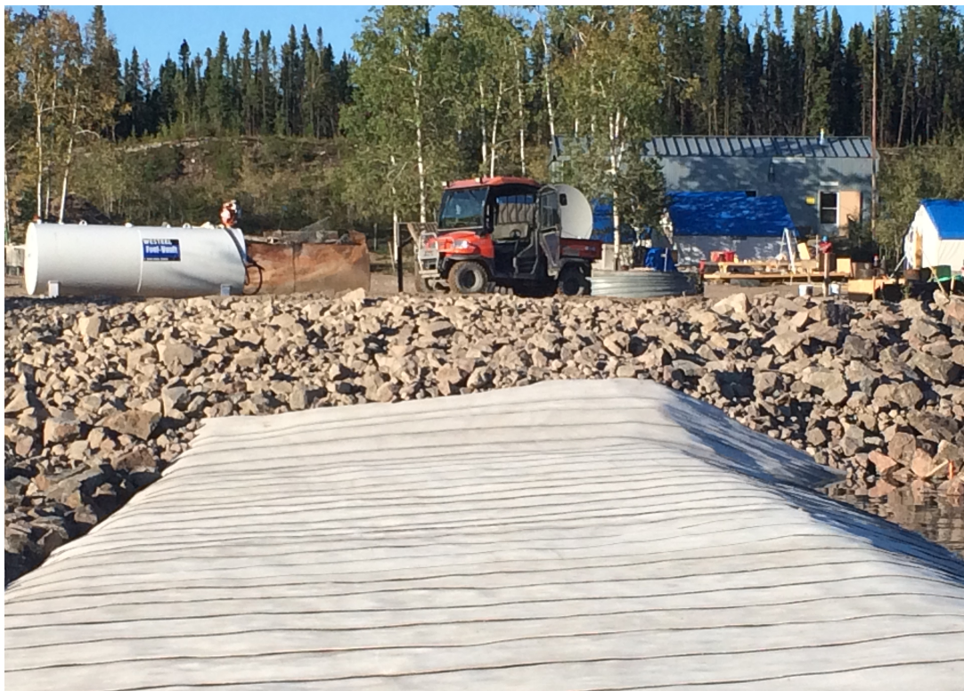
Full view of completed weir
