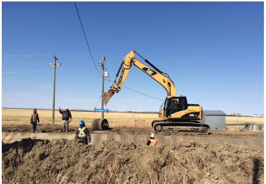
Overhead wires posed an installation challenge
