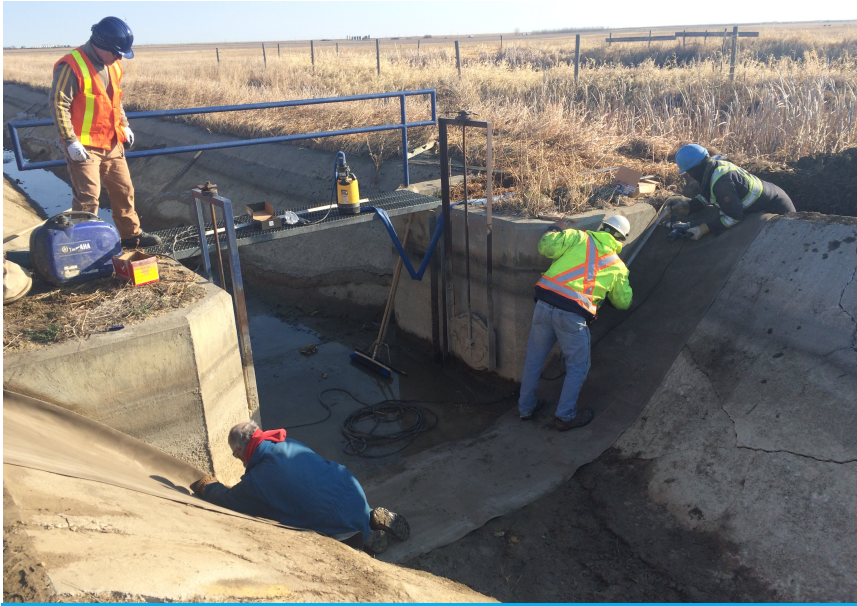
Fixing the first shingle of CC to the old existing concrete
