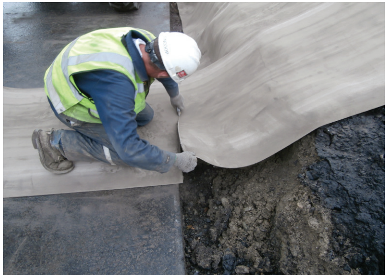
Cutting the CC to length with a utility knife
