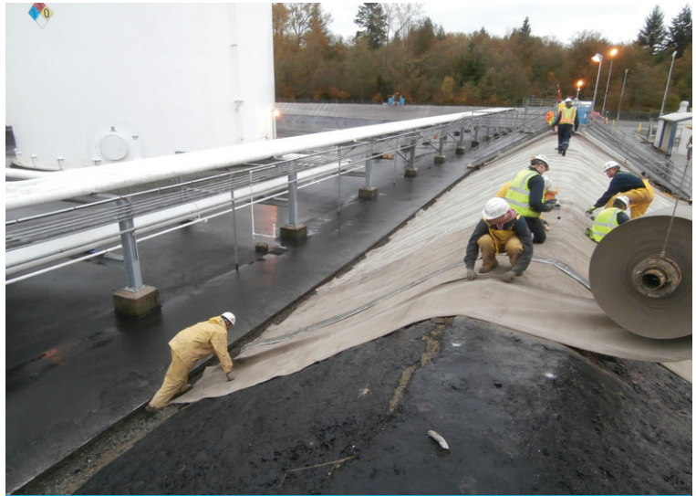
Spooling the CC down the bund
