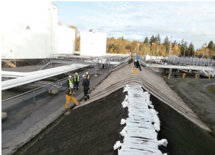
Using sandbags to increase the height of the berm
