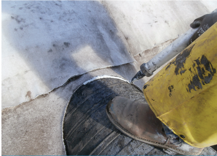
Sealing around piping
