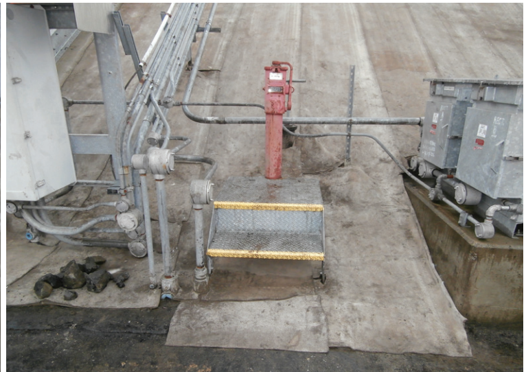
CC accomodating infrastructure
