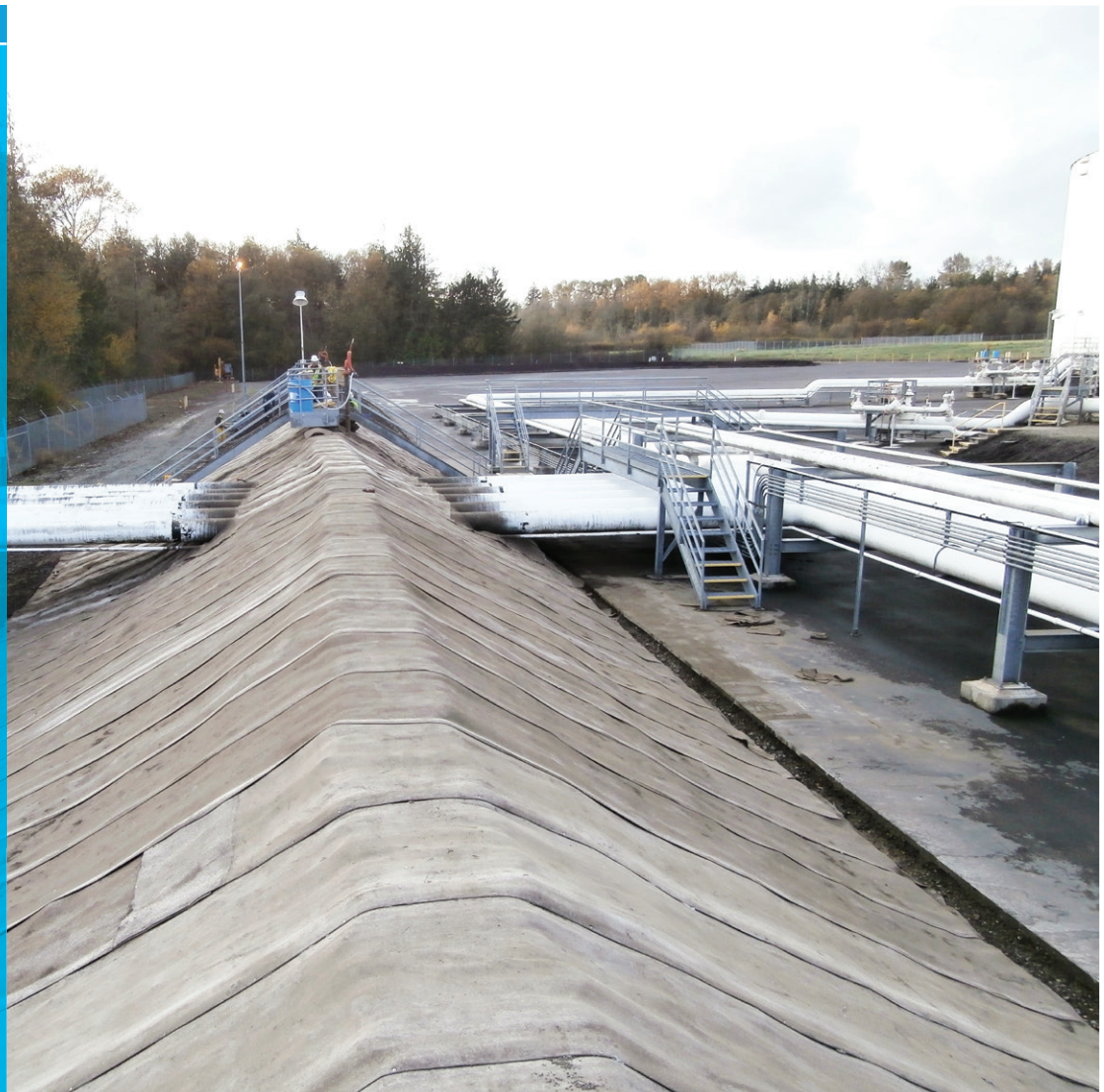
Completed section of bund
