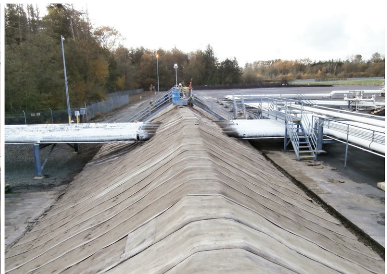
The finished installation
