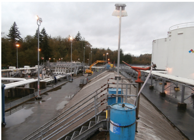
The finished installation
