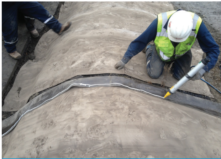
Sealing the overlap with Sika 1-A sealant
