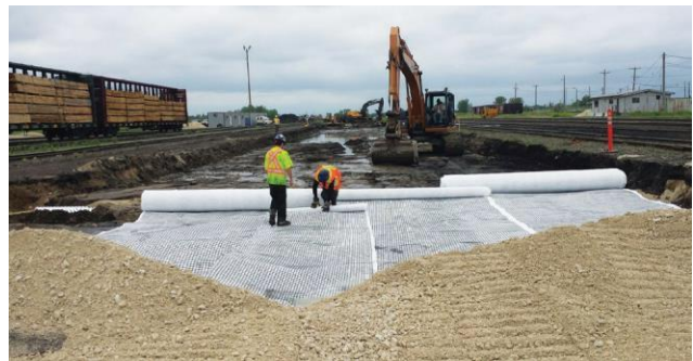
Swamp Grid™ installation in progress
