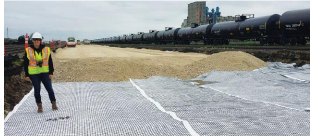
Post-installation showing Swamp Grid™ soil reinforcement performance.
