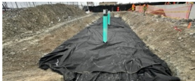
Completed Tank Chamber
