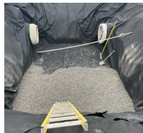
Tank Chamber Before Installation
