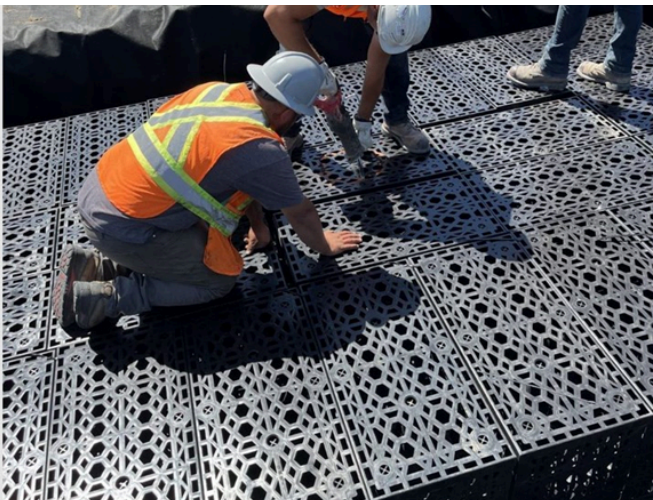
Modules being installed
