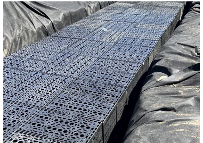
Completed module installation
