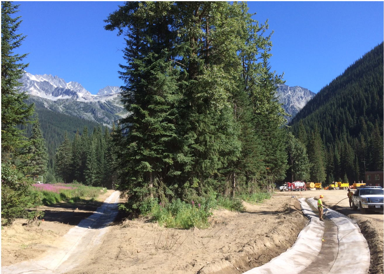
Completed top and lower ditches side by side
