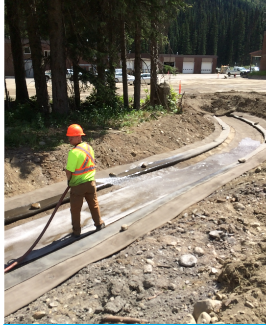
Hydration of lower ditch
