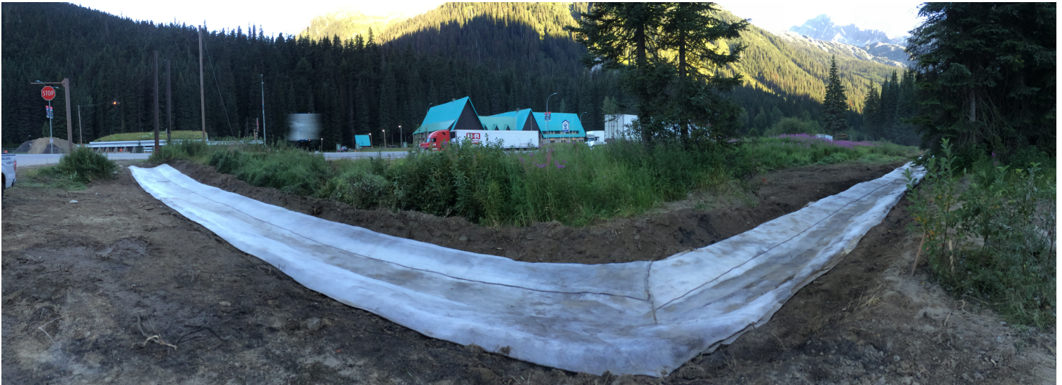
Completed top ditch
