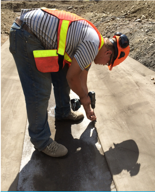
Securing of the CC overlaps
