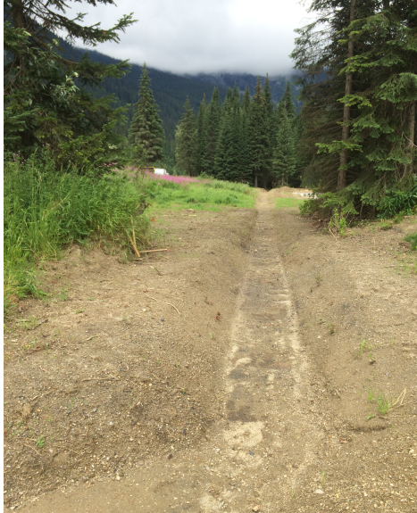
Top ditch - before
