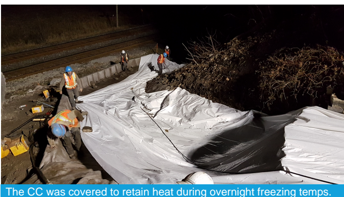
The CC was covered to retain heat during overnight freezing temps.
