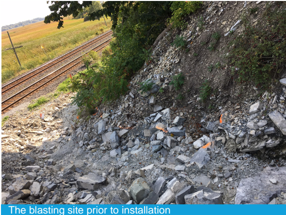
The blasting site prior to installation
