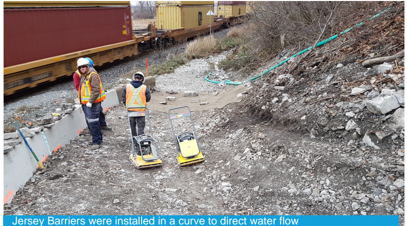
Jersey Barriers were installed in a curve to direct water flow
