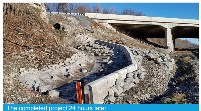
The completed project 24 hours later
