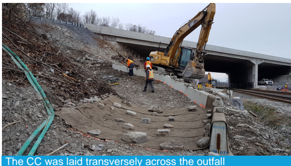
The CC was laid transversely across the outfall
